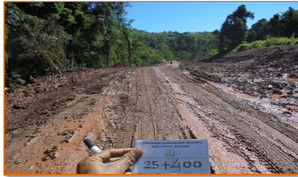
Figure 6: Condition of the Tomata – Beteleme Road Which Is Heavily Damaged.
